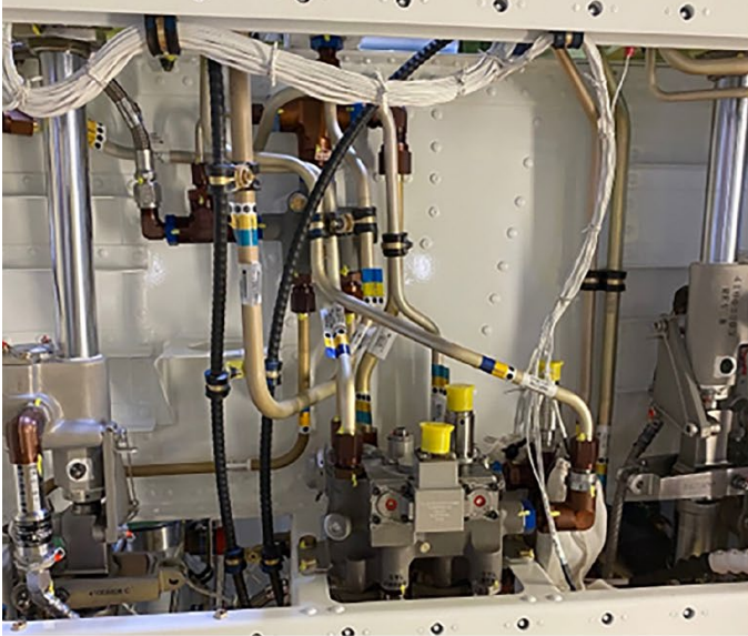
PRE N1 CONTROL RELOCATION VIEW LOOKING AFT
